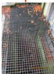
Remove mesh guarding to front elevation lightwells to improve light levels to basement rooms
