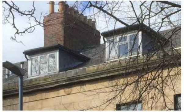
Existing dormers houses 12 & 14 front elevation - to be refurbished and new dormers added to match on houses 4,6,8 & 10
