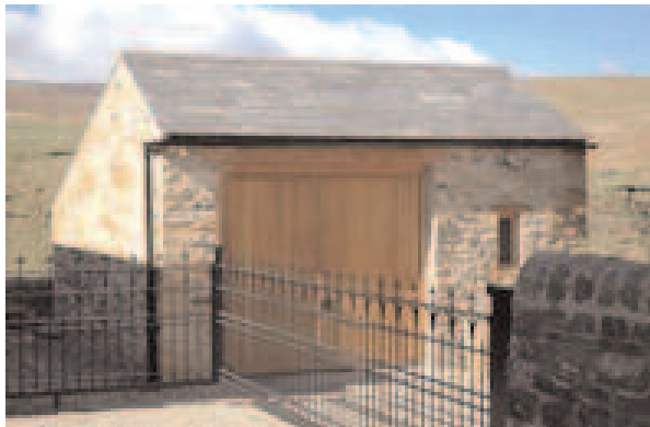
Here a small garage has a simple timber lintel over the door, clearly appropriate use of the inherent properties of timber.
