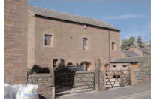
A simple reticent conversion of a Cumbrian barn using existing openings with little loss of character. The retention of boundary walls and gates helps.
