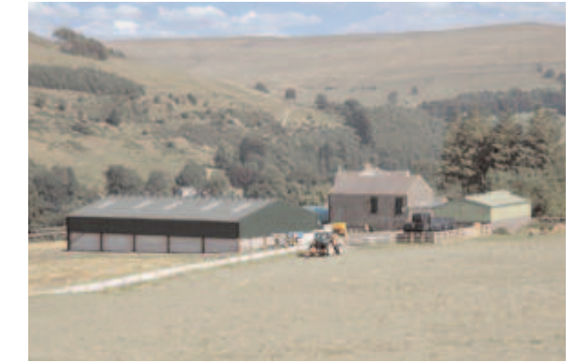
Profiled and coloured sheet material on farm buildings, Upper Teesdale
