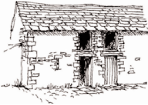
Splitable sandstone roof slates widely used throughout the AONB
