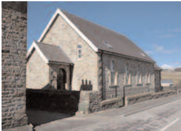
A robust stone porch with a slate roof matching the main roof material and pitch
