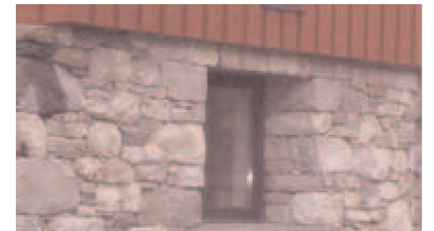
Deeply recessed windows are well protected from wind and rain.
