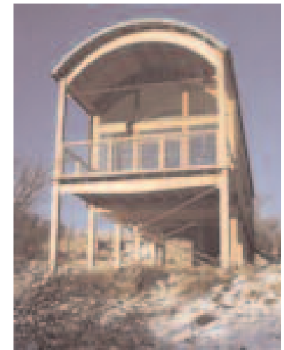
Timber framed home with barn-like roof in profiled sheet and timber cladding
