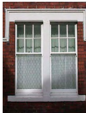
Original timber sash window.
