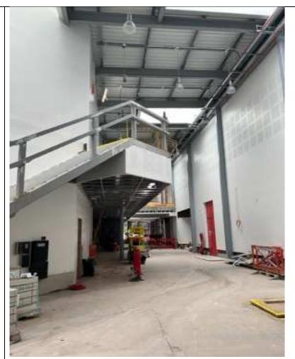
NHS facility now advanced to installation of flooring, sanitary wear and ICT / Electrical points.
