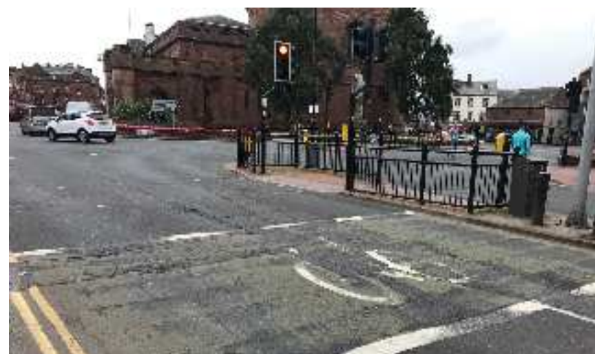
Advanced cycle stop box on Botchergate, heading to English St.
