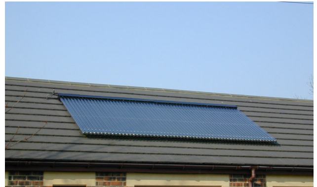
Fig 96. Evacuated tube solar water heating.
