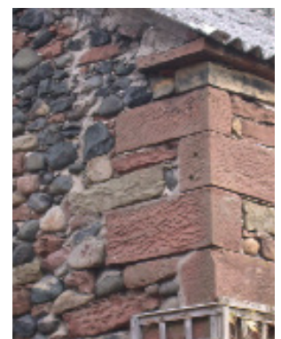
Fig 62. Cobble walls and stone quoins, Dalston
