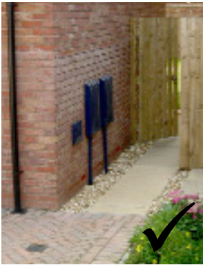
Fig 63. Meter boxes should be mounted discreetly and not on the main elevation. Sunken 'in ground' boxes are also available.
