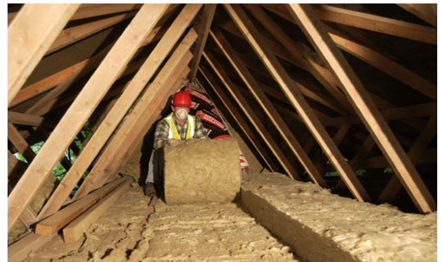
Fig 94. High levels of insulation is one of the key components of a sustainable building. 270mm of insulation is currently recommended. Energy Saving Trust
