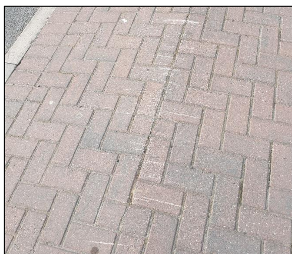
Scratch marks on the speed hump
