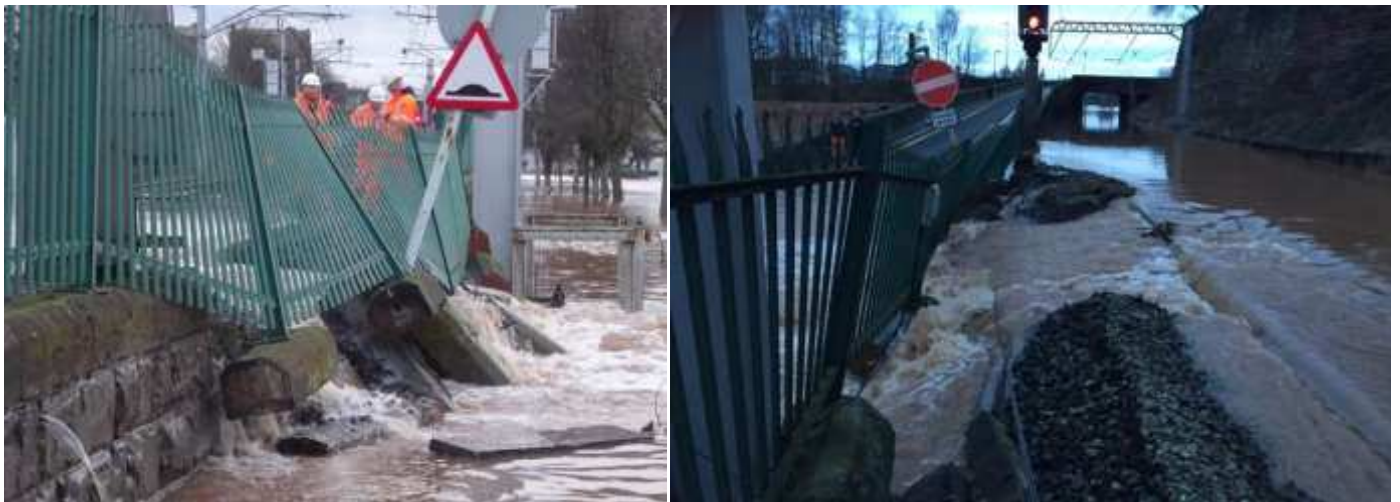
Figure 21 Wall along railway at entrance to Viaduct Estate that collapsed during the flood event
