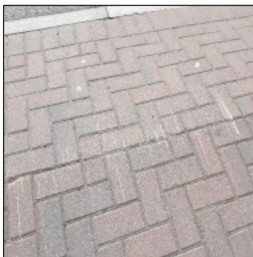
Scratch marks on the speed hump
