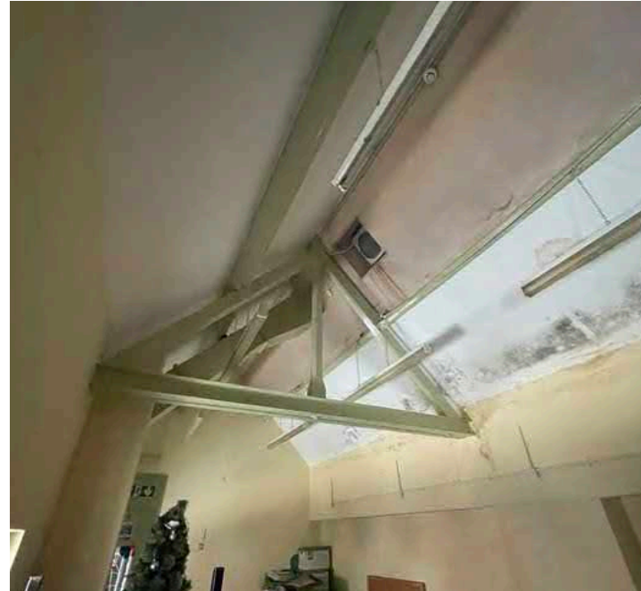
Areas of damp appearing at roof level in upper floors.
