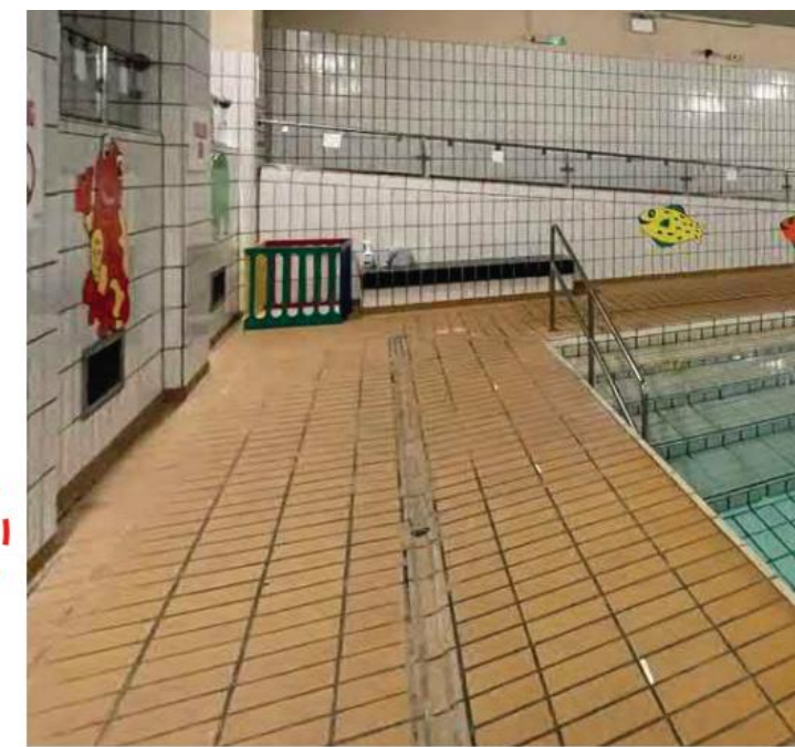
3. Draining floors to be made level and covered in suitable slip resistant fire retardant surface.
