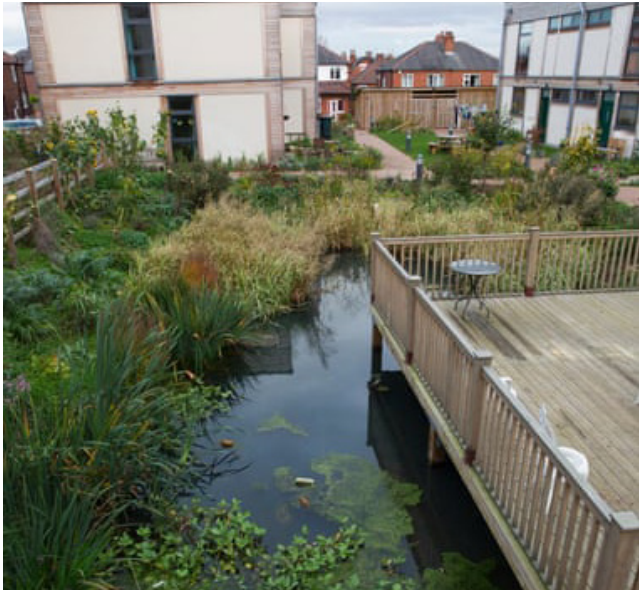
Fig. 42 Lilac Grove, Leeds. Shared green spaces between houses serve as natural filter and storage tanks for water reuse.
