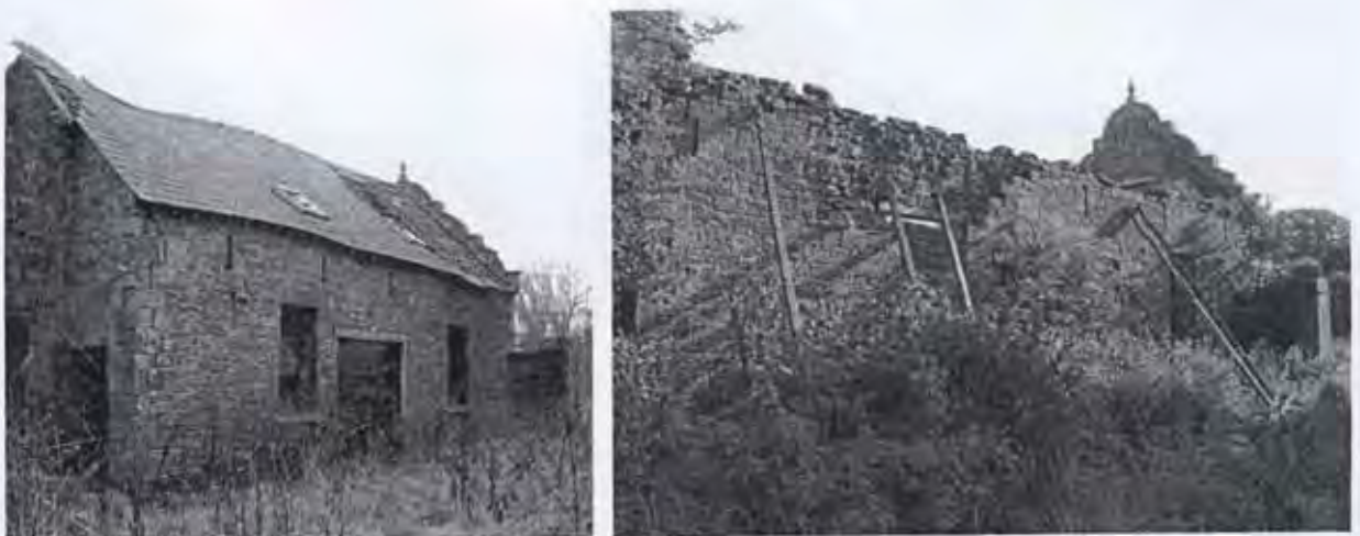
Fig. 21 & 22 - Coach House November 2007 - Coach House May 2008 Showing collapse of wall and roof following theft of stone lintels
