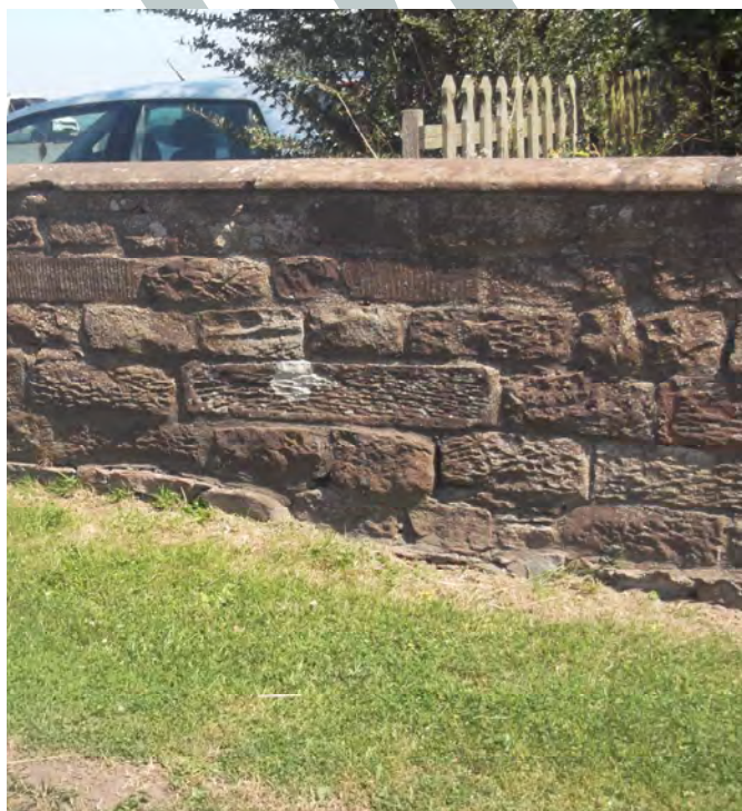
Figure 24: Reused lintols in stone boundary walls
