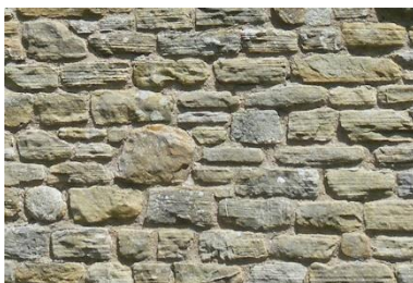
Figure 23 Buff roughly dressed coursed sandstone; mixed red and buff sandstone; and roughly- tooled and dressed ashlar walling
