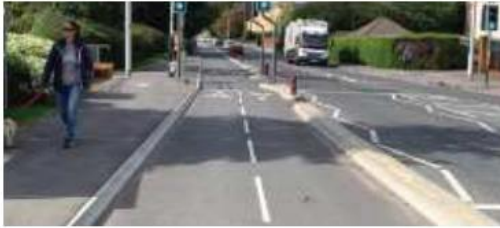
Two way segregated cycleway.
