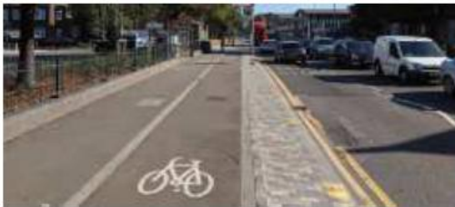
On road segregated (stepped) cycleway.
