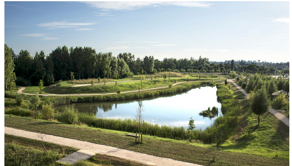
Fig. 41 The attenuating pond at Sutcliffe Park, London. A park focal point which provides an ecological habitat whilst managing water from the nearby development.
