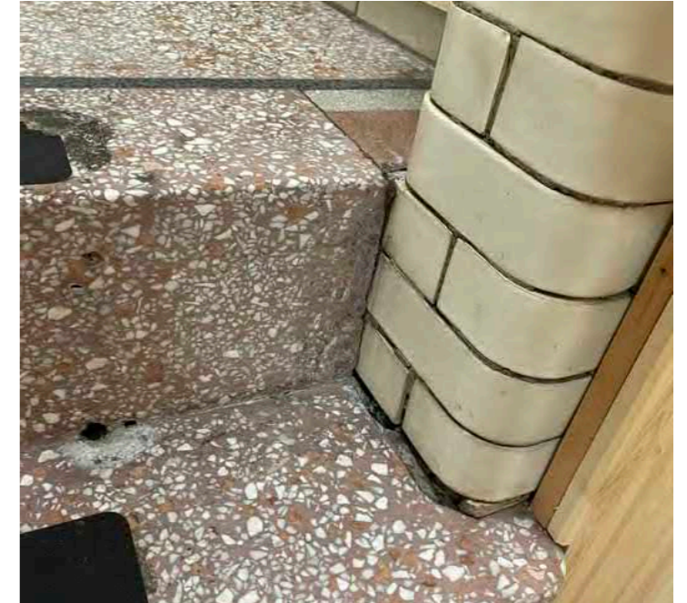
Areas of presumed original terrazzo flooring.
