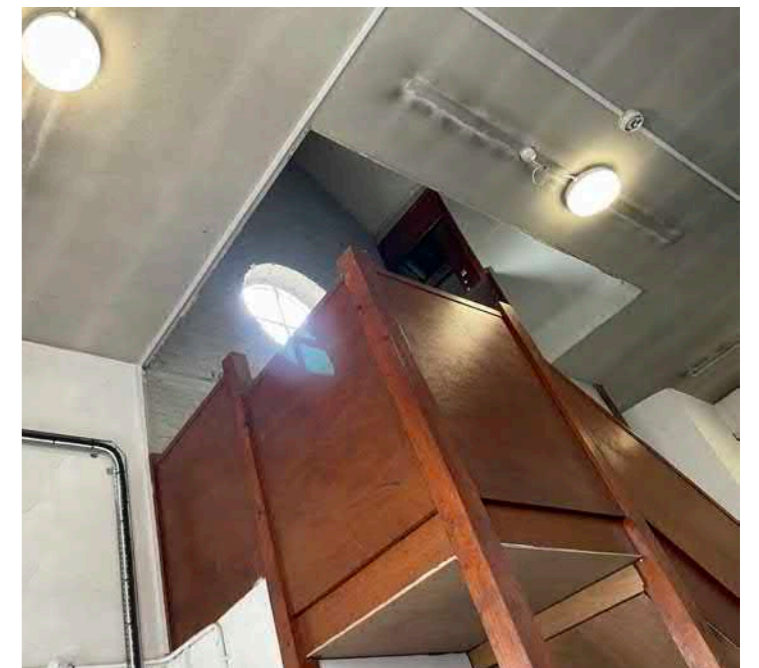
Timber clad access stair to roof / loft space from staff areas.
