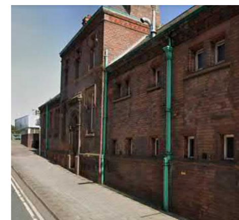
Red brickwork to external facades
