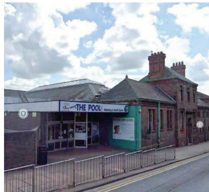
Figure 72: Existing 1970's lobby and principal elevation of the James Street Baths.
