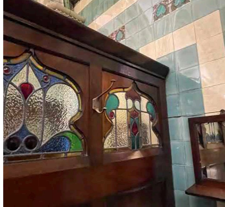
Existing decorative changing room dividing screens and associated wall hung fixtures.
