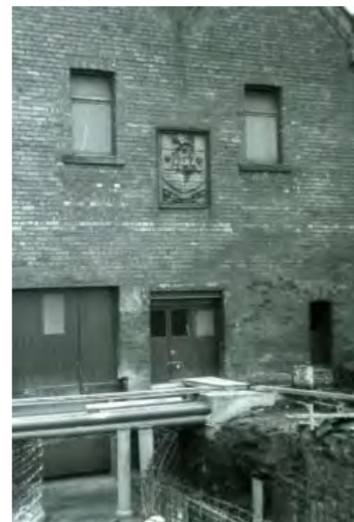
Figure 10: James Street Baths, c.1974. Foundations of new baths in foreground. Cumbria Image Bank. ref: ct08095
