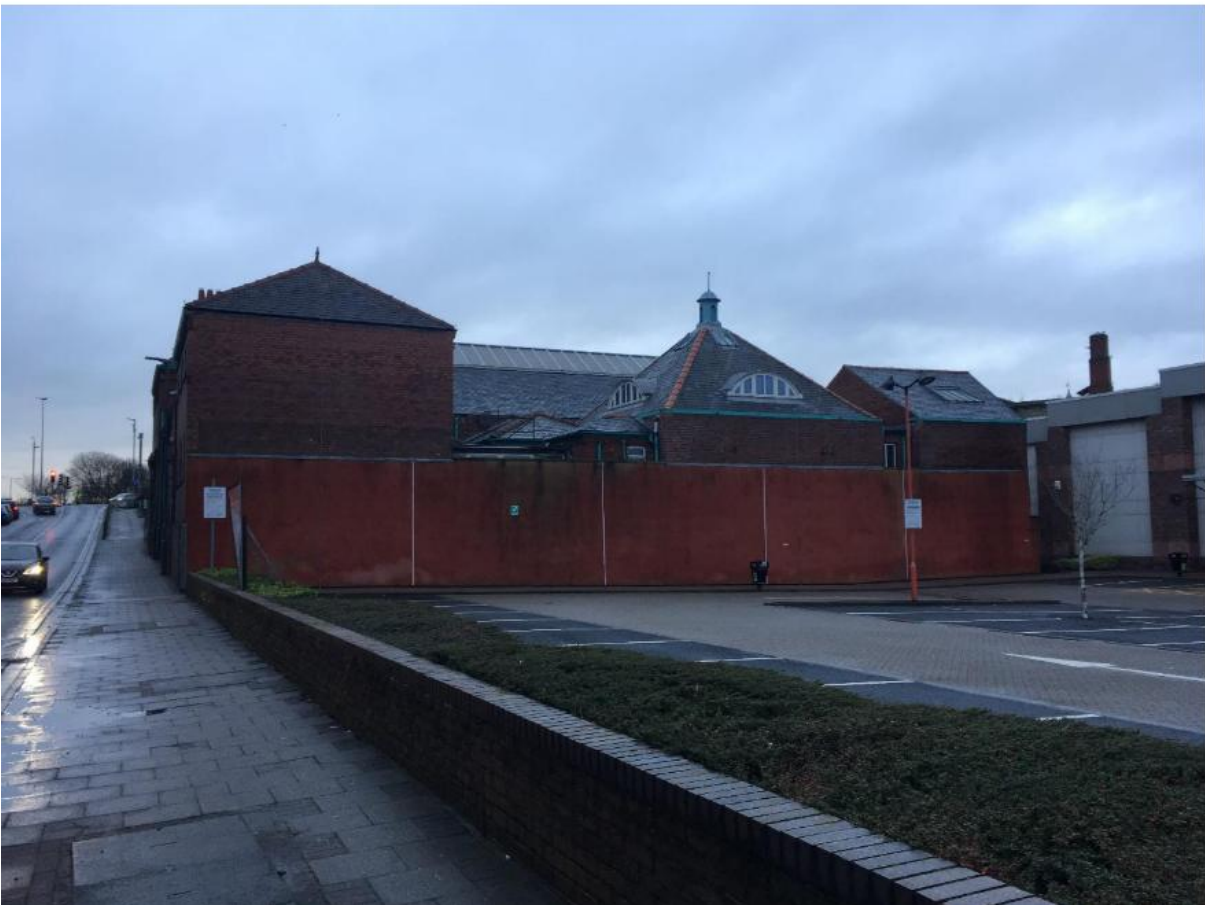
Fig.59 Below: South elevation which formerly abutted the metal box manufactory
