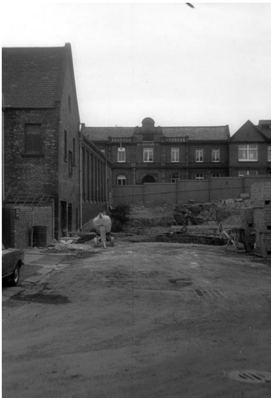
Fig.30 Above: Photo circa 1970 looking towards James Street
