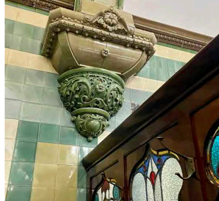
Decorative glazed wall tiling, corbels and arch features.
