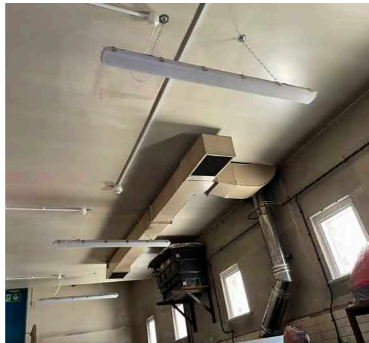
Double height wash room.
