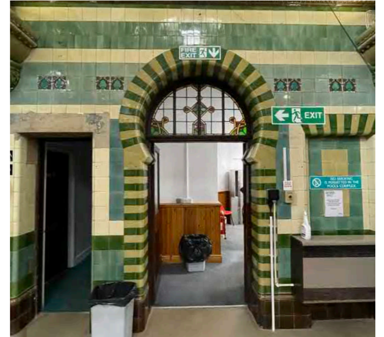
Decorative glazed wall tiling and arch features - looking towards the low-quality finishes of the entrance area and locker room.
