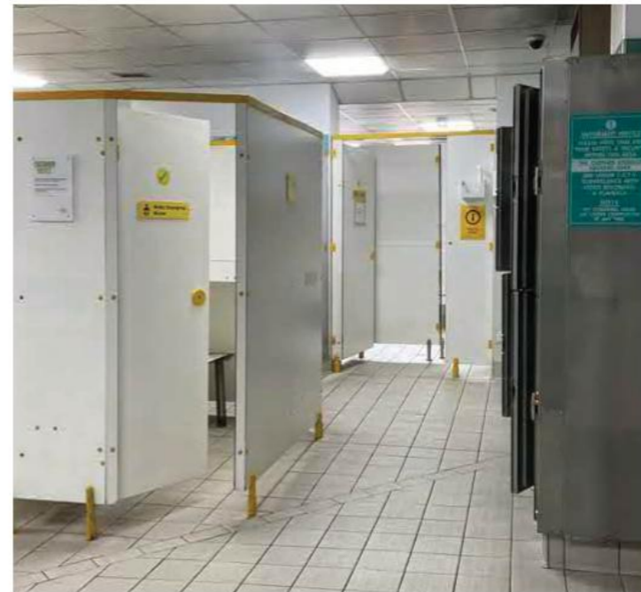
5. Changing room fixtures to be removed.
