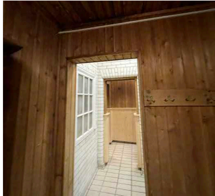
Areas of existing glazed tiling. Sauna/ hot room areas lined within poor quality and degrading timber.
