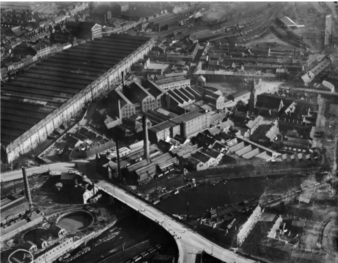
Fig.15 Below: Aerial from Britain from Above of the Railway Station & Factories on James Street 1928, (ref: EPW025040)
