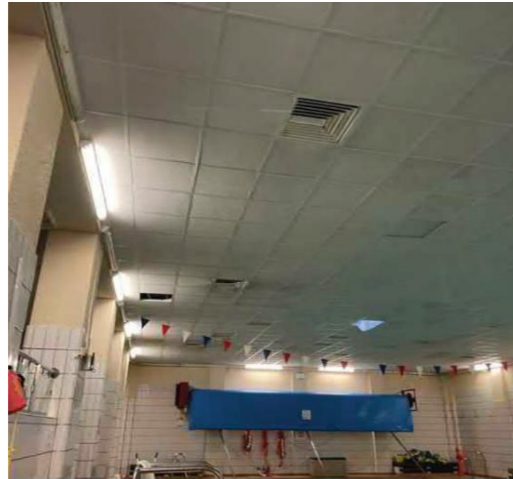
1. Suspended ceiling removal over 20m main pool.
