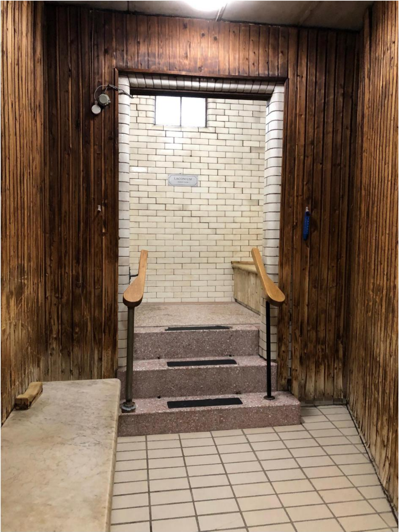
Fig.42: Interior showing hot rooms no. 2 and no. 3 (dated 2019 before the timber t&g was replaced)
