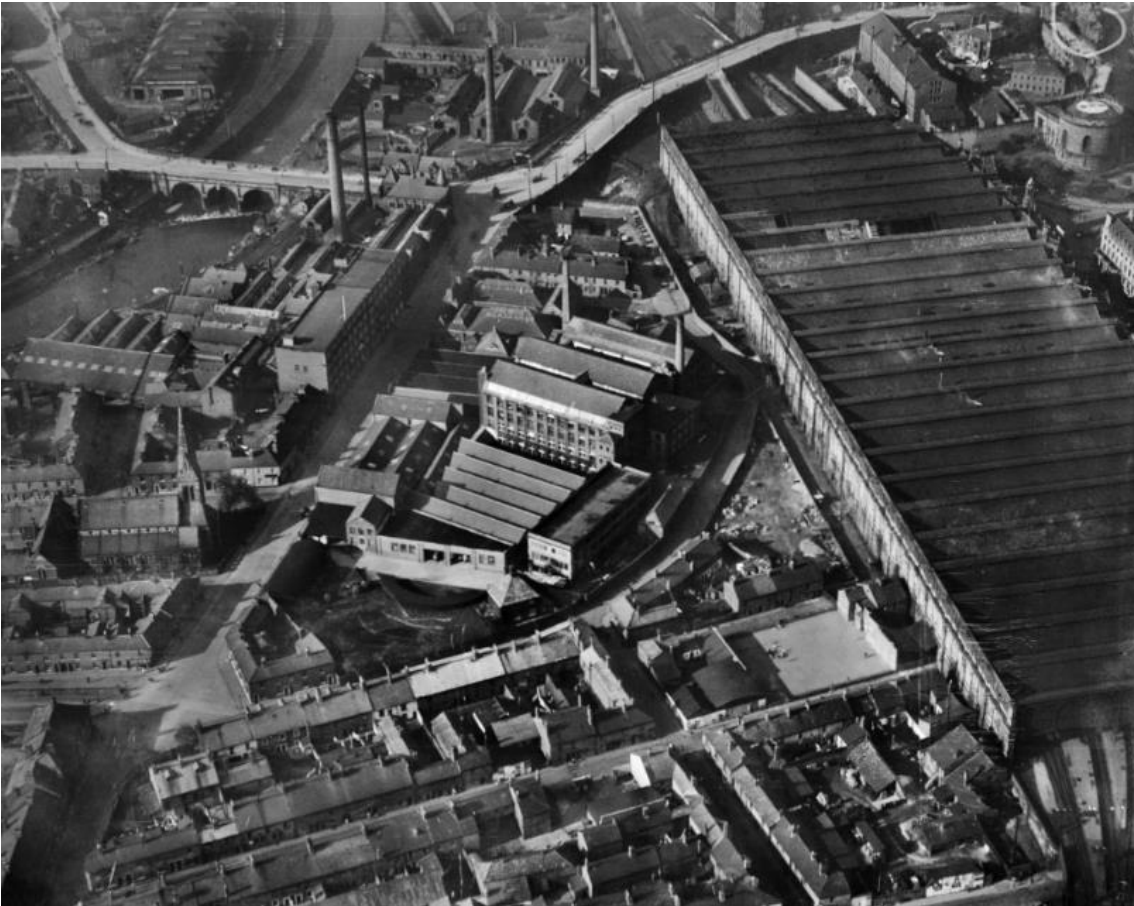
Fig.14 Above: Aerial from Britain from Above of the Railway Station & Factories on James Street 1928, (ref: EPW025039)
