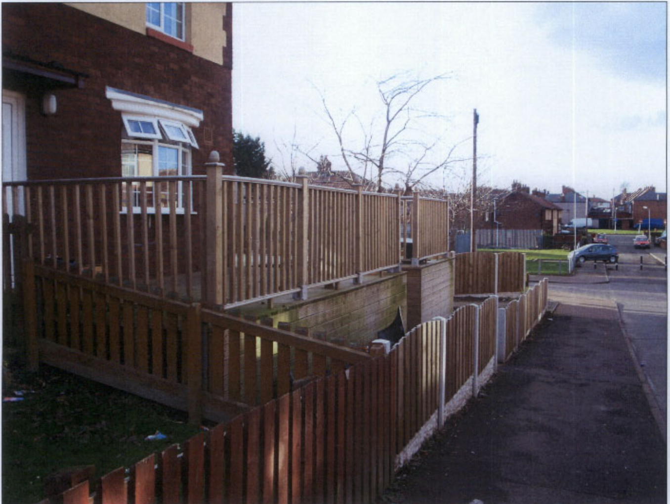
Photograph 3: Photograph of No 3 Dowbeck Road taken from outside the adjoining semi detached dwelling looking down Dowbeck Road. Members will note the decking is as refused by committee on 11/7/08 under application reference 08/0337.
