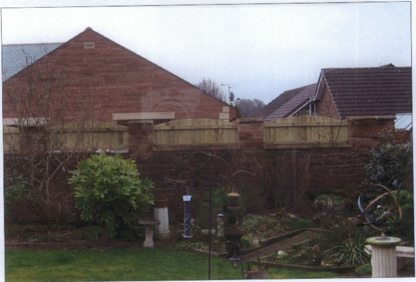
Photograph 3: A more detailed photograph that illustrates the coursed sandstone that has been used on the construction of the stone pillars, which face inwards towards the garden of Spring Grove.
