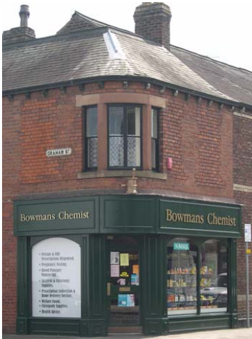
Attractive shopfront with individual mounted lettering and a restrained colour scheme.
