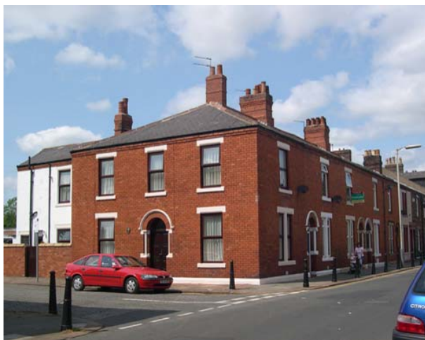
Red brick terraces of Denton Holme, often with substantial stone cills and lintels over doors and window openings.
