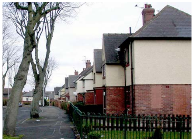
Sheltering, overhanging eaves and Arts and Crafts/garden suburb design are typical of inter-war housing such as at Longsowerby.
