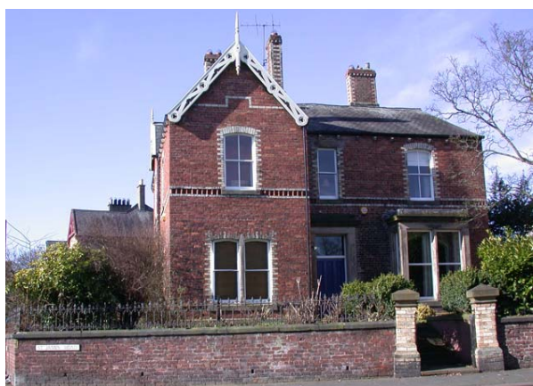
Villa on St James’ Road with decorative brickwork, ornate bargeboards and central finial.
