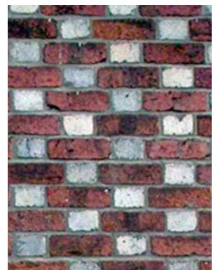
Flemish bond brickwork adds to local distinctiveness.
