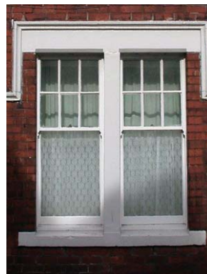
Original timber sash window.
