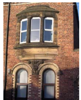
Decorative brickwork and an unusual oriel window on the first floor.
