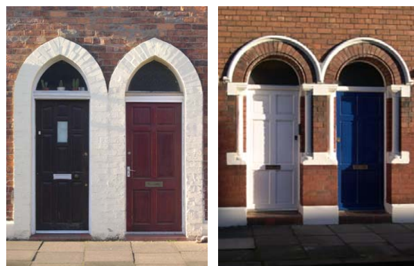
Brick gothic arch adding interest to simple terrace.
