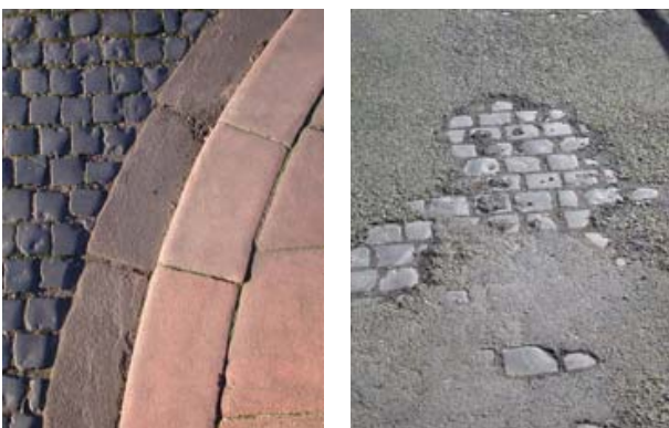
Stone setts and cobbled lanes are characteristic of Denton Holme. These are high quality and expensive surfaces which should be maintained and enhanced. Where covered in tarmac this can be readily re-exposed.
