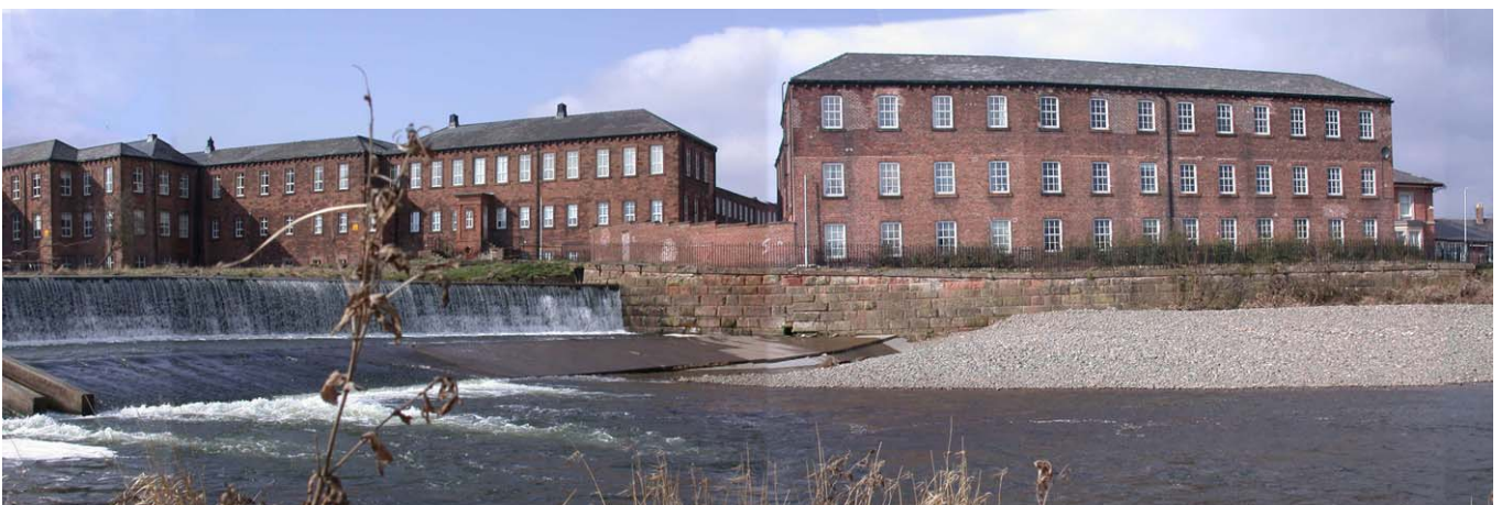
The former mill and weir at Holme Head. The mill has been converted to residential use.
