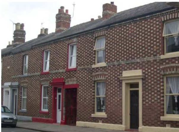
Use of contrasting flemish bond brickwork is a strong local tradition in Carlisle. Its simple pattern creates visual relief on sometimes large expanses of wall. Norfolk Street.
