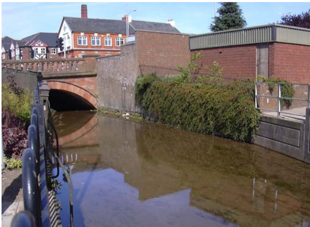
Millrace on the Little Caldew. New development should front on to these distinctive features, maximising their value as townscape assets.
