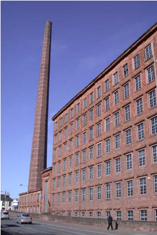
Shaddon Mill and its landmark Dixon's Chimney.
