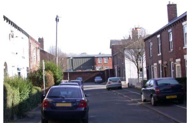
A quirk of historic development is the occasional abrupt termination of streets. These frustrate legibility and should be resolved when sites come forward for redevelopment, reconnecting sites to adjacent street networks.
