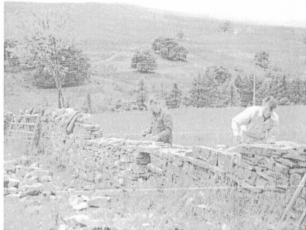
"Traditional skills such as drystone walling need to be retained" – © Janet Elliot.
