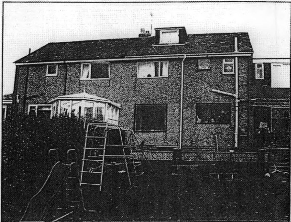
Photograph 1: Photograph of the rear of No.4 Holme Close, Scotby, which illustrates the position of the conservatory to the rear of No.3 Holme Close.
