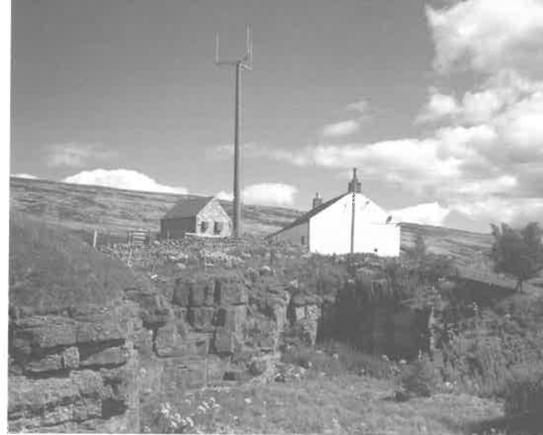
"Telecom mast – Teesdale" – Charlie Hedley © Countryside Agency.
