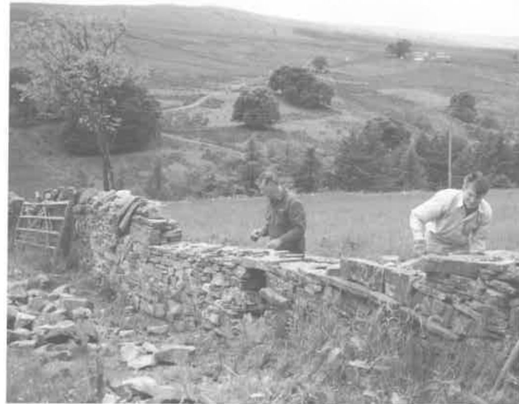
"Traditional skills such as drystone walling need to be retained".
