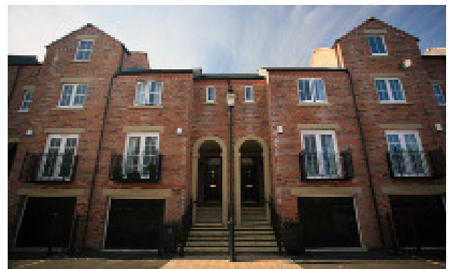
Fig 53. Terraced housing drawing on the terraced pattern typical to Denton Holme but providing for undercroft parking and flood resilience. C Storey Homes.
