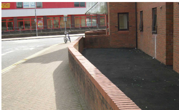
Fig 17. Ill considered outdoor space of no practical or aesthetic value. In addition, impermeable surfaces contribute to surface water run off and increased flood risk.
