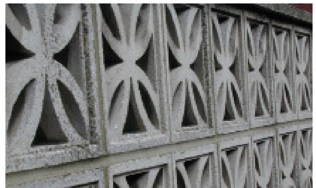
Fig 40. Breezeblock walling is unlikely to make an appropriate boundary treatment in areas visible to public view.
