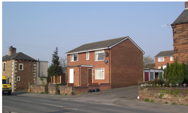
Fig 50. Infill development which fails to take note of the materials, form, proportions or position in relation to the frontage of its neighbours.
