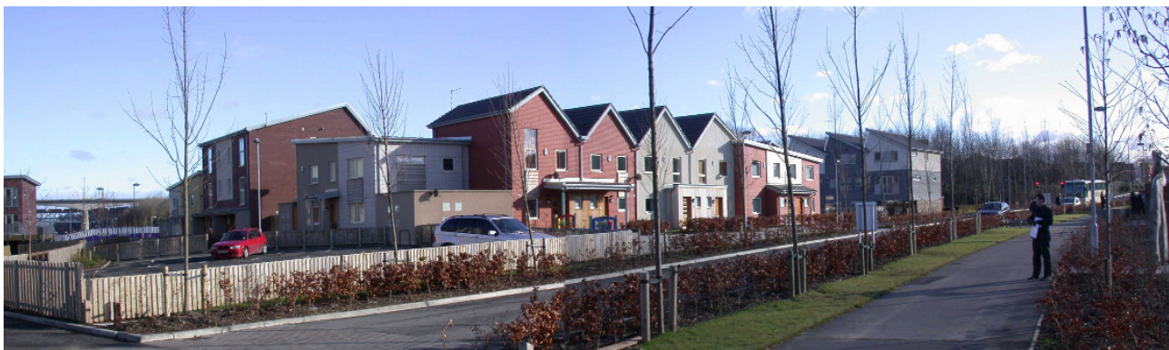
Fig 68. A variety of dwelling sizes in a contemporary style, Taylor Wimpey development, Gateshead.
