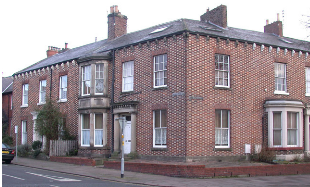
Fig 43. Double-aspect corner building providing ‘eyes on street’ Howard Street, Carlisle.
