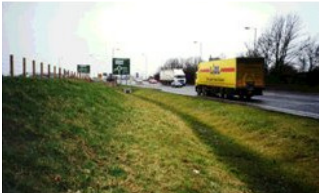
Fig 28. SUDS incorporated into a new highway as an infiltration swale, minimising the burdening of drainage systems.
