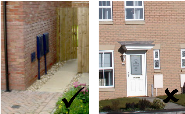
Fig 63. Meter boxes should be mounted discreetly and not on the main elevation. Sunken 'in ground' boxes are also available.
