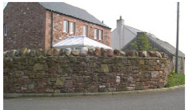
Fig 33. A new random rubble boundary wall in local sandstone appropriate to rural Cumwhitton.
