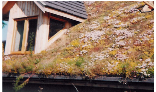
Fig 98 'Green', sedum roof, providing wildlife habitat, slowing rainwater run-off and providing additional insulation.
