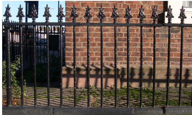
Fig 36. Cast iron railing typical of Carlisle's Victorian terraces. Hawick Street.
