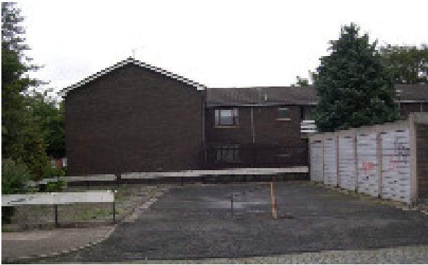
Fig 44. Blank Facade and poorly overlooked parking which invites antisocial behaviour, Denton Holme.
