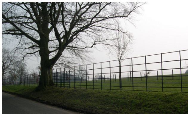
Fig 38. Estate fencing can be an effective and cost effective boundary treatment.
