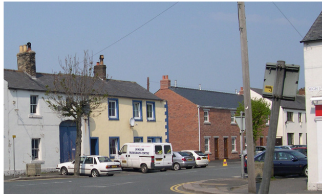
Fig 67. An infill development which respects the plot position and scale of its neighbours. A rendered finish would match neighbours better.
