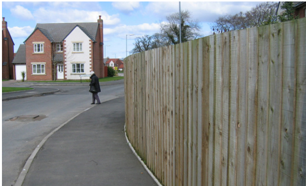
Fig 35. Blank fencing should not usually abut footpaths. A brick wall or piers with dwarf wall, infilled with railings would be a better treatment for this boundary.
