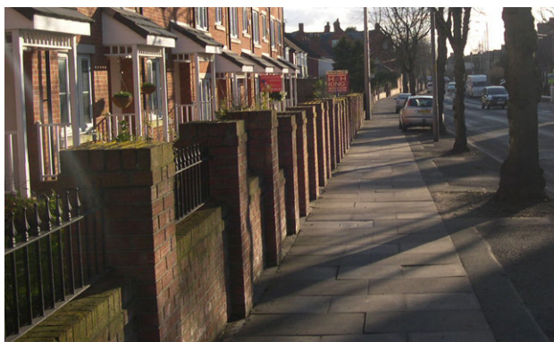
Fig 41. New boundary at Dalston Road creating a robust demarcation of public and private space.
