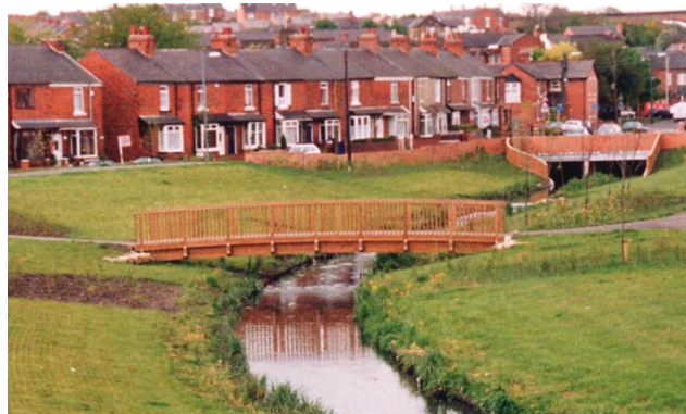
Fig 32. The above, following works to return the watercourse to its natural open channel at the centre of a public park.
