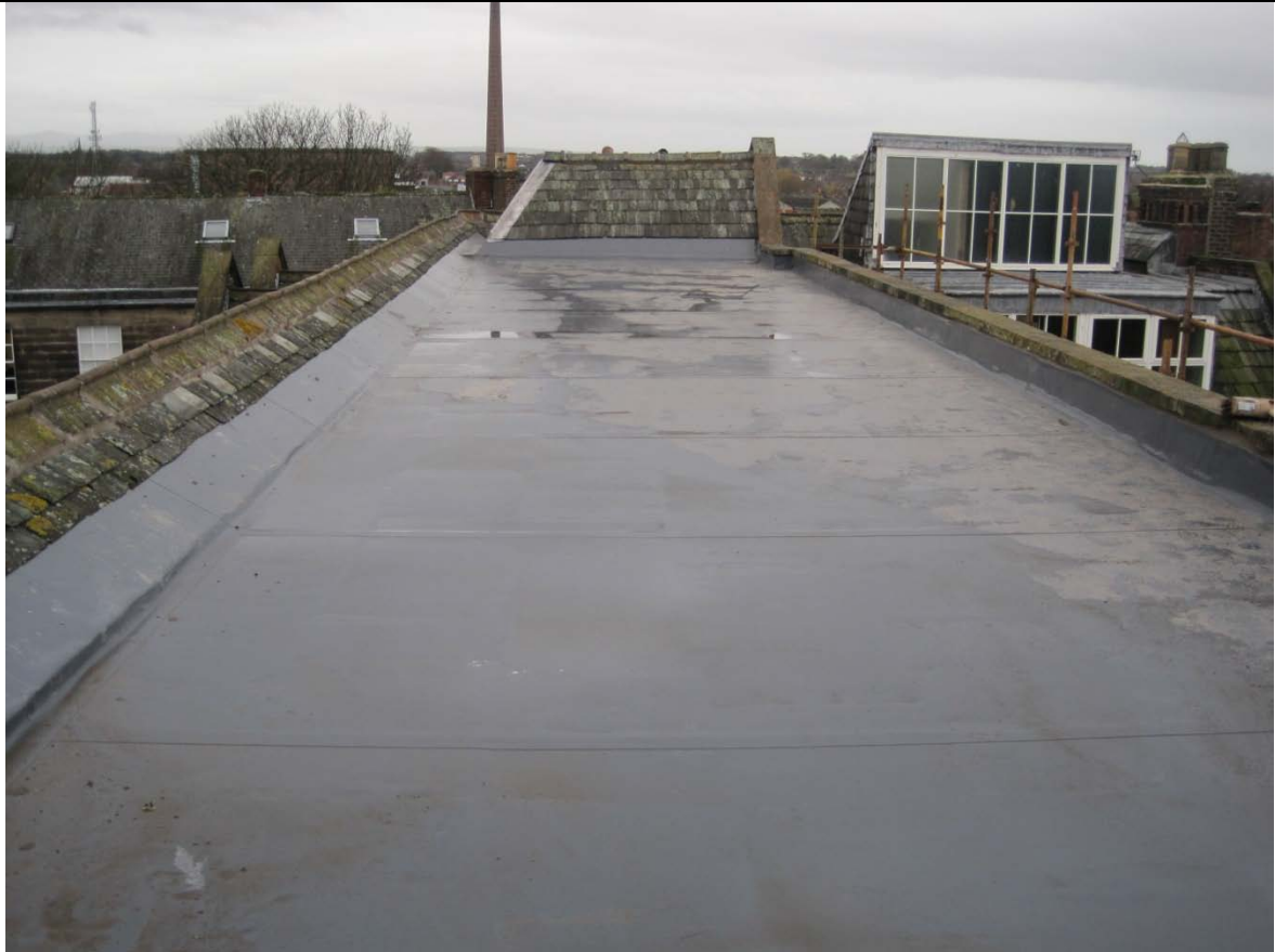
AFTER – Looking south
