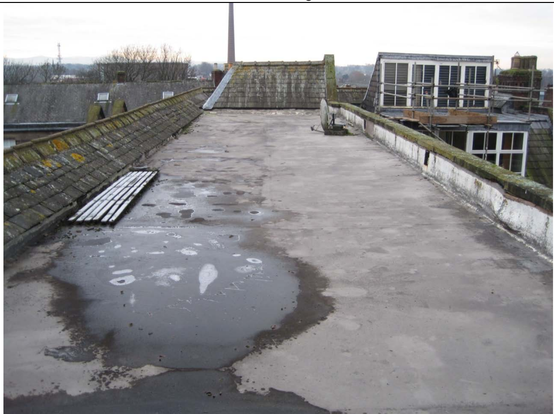
BEFORE – Looking South
