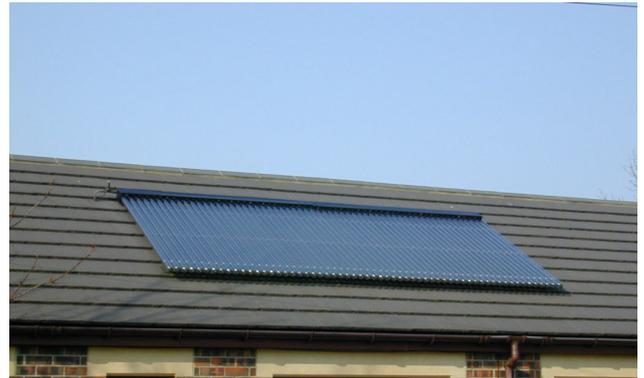
Fig 96. Evacuated tube solar water heating.
