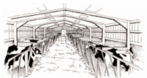
Interior of a typical modern farm building showing shallow roof pitch and portal frame construction
