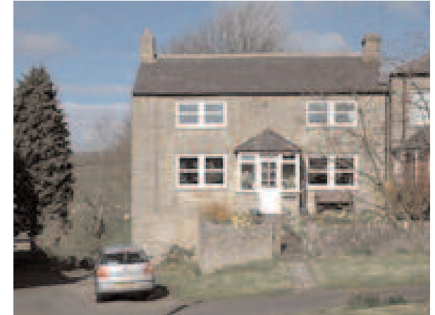
Oddly proportioned replacement windows give the house a squashed appearance
