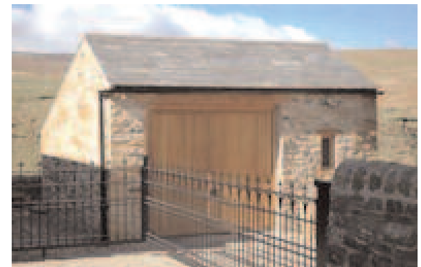
Here a small garage has a simple timber lintel over the door, clearly appropriate use of the inherent properties of timber
