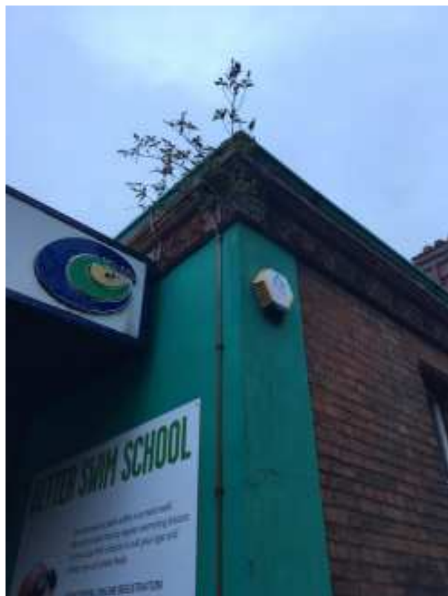
Fig.54 Below Left & Fig.55 Below Right: Vegetation growth
