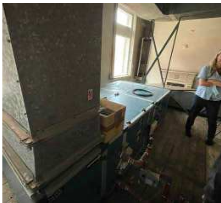
Swimming pool extract duct in upper floors.
