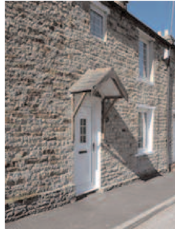
A neat canopy over the door avoids obstruction to the pavement
