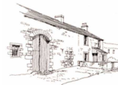
Longhouse from the 18th century; Dufton. The original entrance to the house through the byre has been blocked up and a later door and porch added to the house itself
