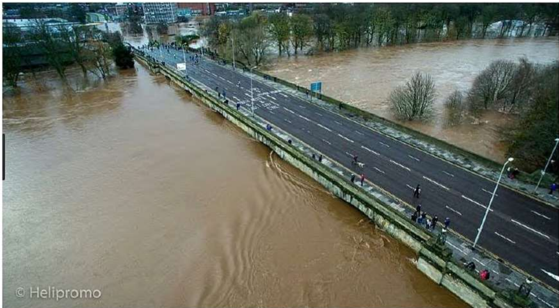
Figure 6 Upstream view from north bank – eye witnesses maintain there is a 2m – 3m differential to the downstream side not 200mm as contended by the EA modelling
