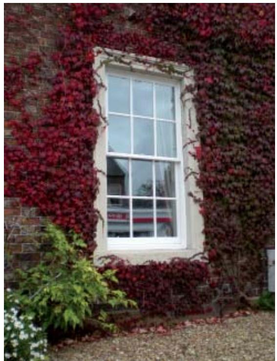
▲ New timber vertical sliding sash window with dimensions to match the original joinery.
