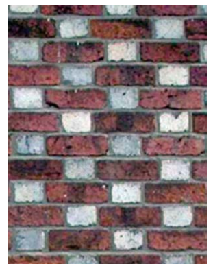
Flemish bond brickwork adds to local distinctiveness.
