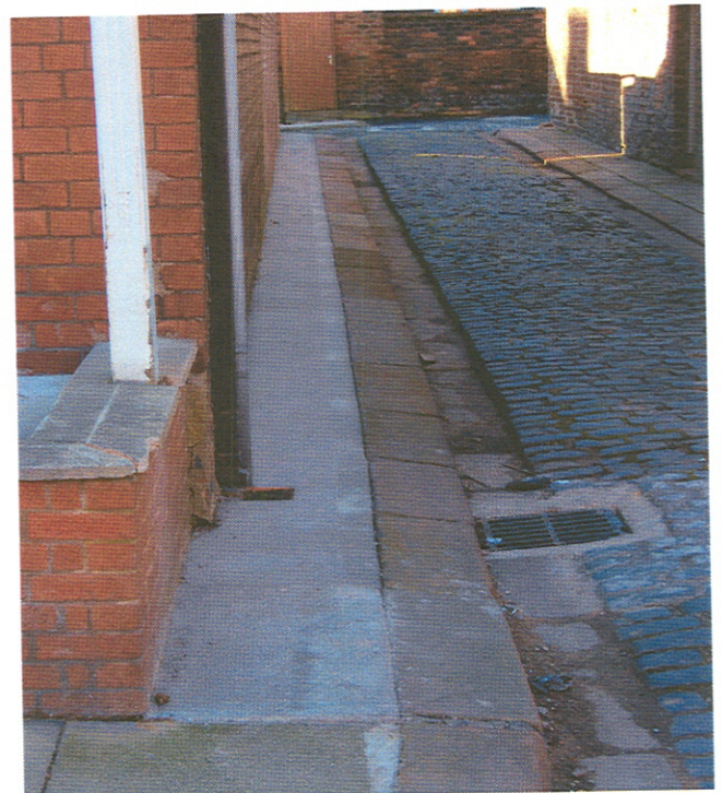
Side of 22 Tullie St
