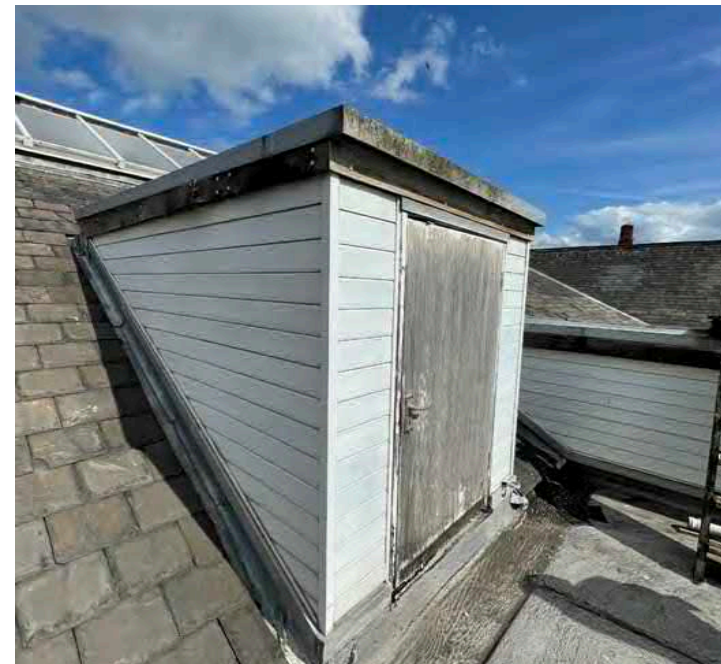
Poor quality roofscape additions, access hatches etc.
