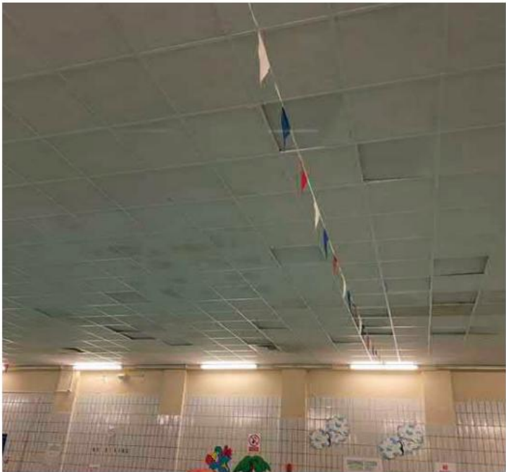
Suspended grid in-lay ceiling above the large/main (20m) pool showing signs of age
