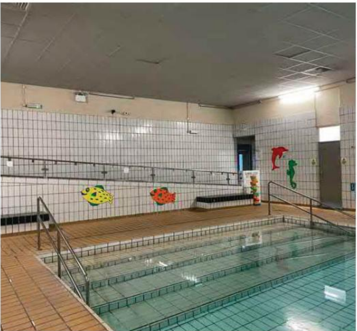
Suspended grid in-lay ceiling above the small (10m) pool showing signs of wear and deterioration
