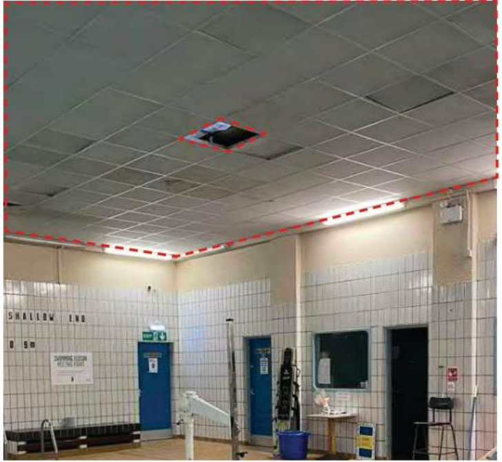
Suspended grid in-lay ceiling above the large/main pool ceiling tiles missing or damage/ lifting
