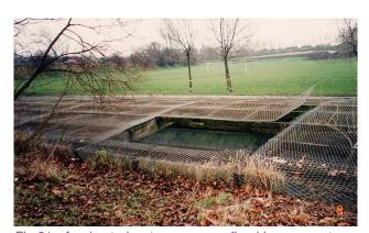
Fig 31. A culverted watercourse confined in a concrete channel with a mesh cover, Cong Burn, Chester-le-Street.
