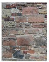
Fig 61 Dressed rubble sandstone walling, Stanwix.
