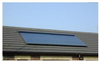
Fig 96. Evacuated tube solar water heating.
