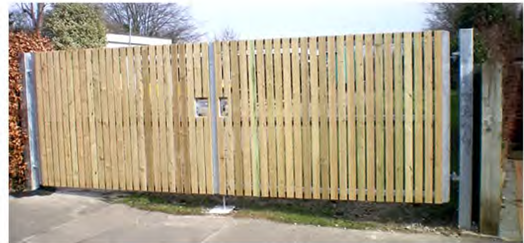
c 6ft high timber palisade double security gates on galvanised steel frame
