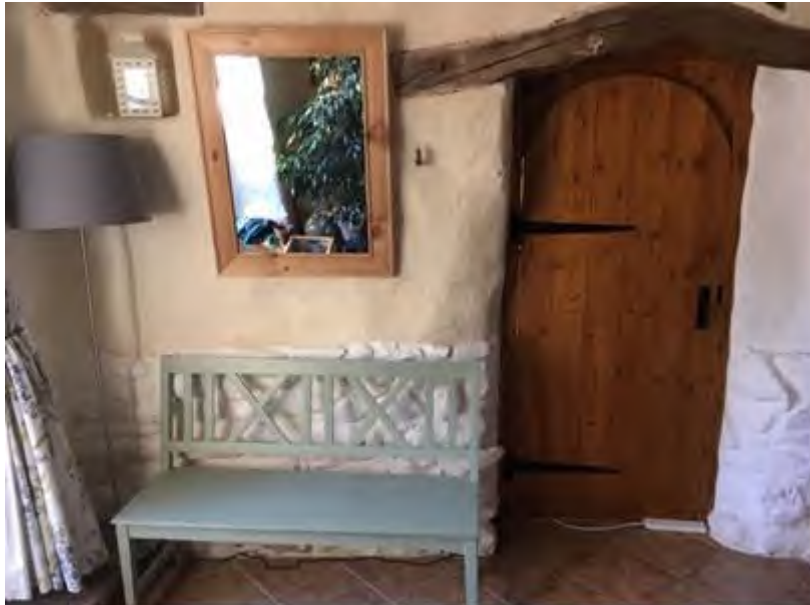
Photograph L - Internal clay daubin taken from inside the living room (door into kitchen)
