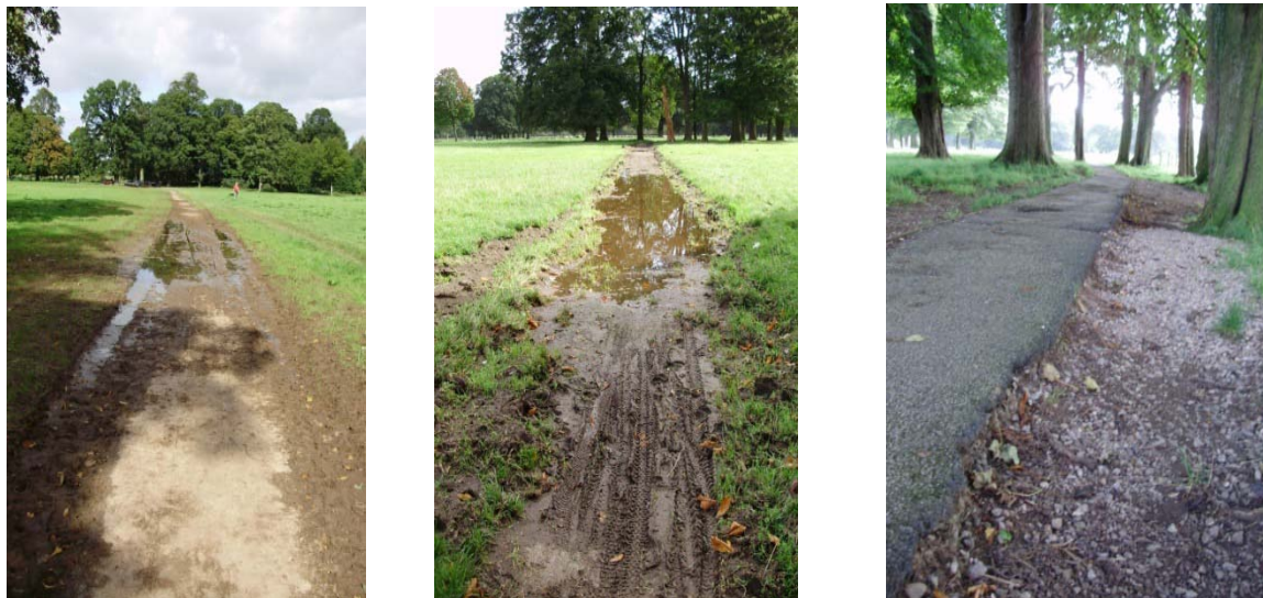
Drainage issues on Hadrians Wall National trail Resurfacing needed on footpath to cenotaph Flood damage on riverside footpath
