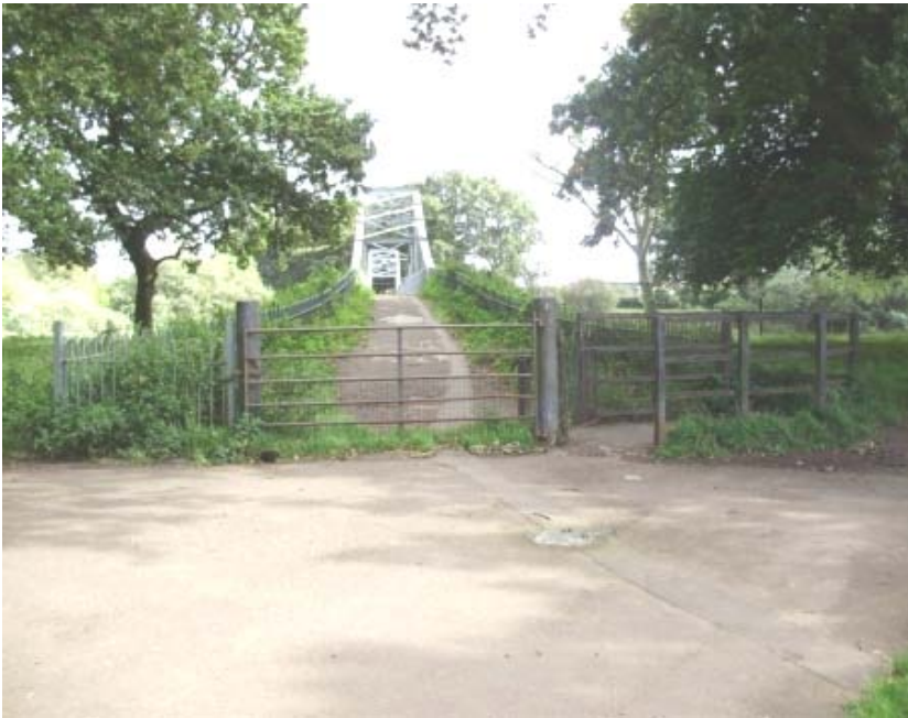
Figure 11. Memorial Bridge – The gates will be replaced with the new kissing gate design, fitted with a ‘Radar’ locking device to allow easy access for people with a disability or with a disability scooter.
