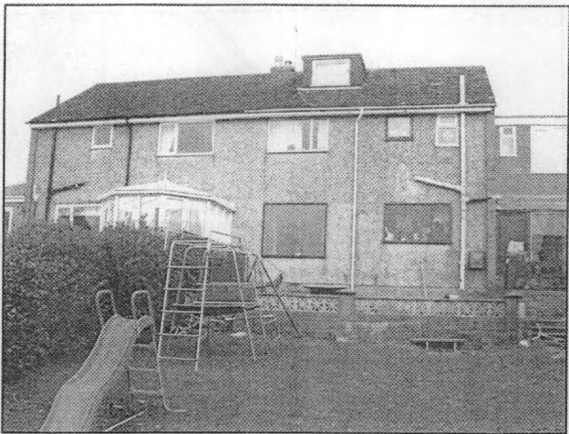
Photograph 1: Photograph of the rear of No.4 Holme Close, Scotby, which illustrates the position of the conservatory to the rear of No.3 Holme Close.
